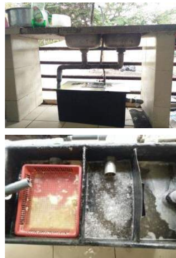
Figure 2.1 The modified oil trap system design.
