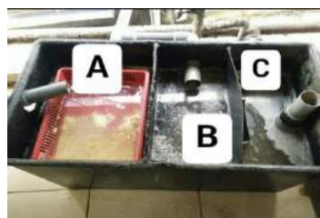
Figure 3.1 Oil trap system configuration with three storage compartments of A, B and C.
