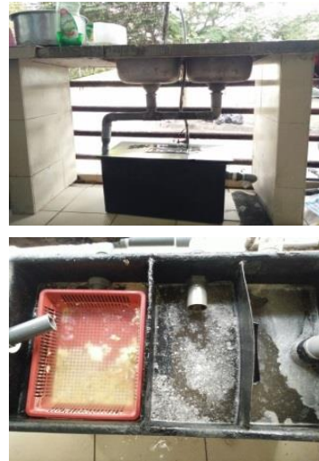
Figure 2.1 The modified oil trap system design
